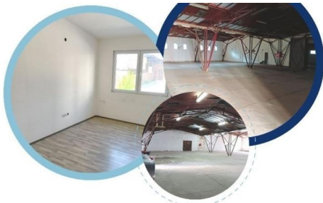
MAGACINSKI PROSTOR 1420M 2 - RAMPA 0677/000-222
